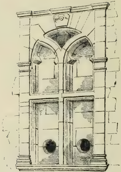
FIG. 1514.—Ballingry Church. Window in North Aisle.
